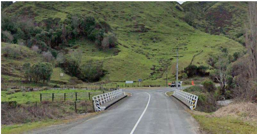
Figure No. 5.3 – Bridge 8: Te Anga Road (Source: Google Earth)
