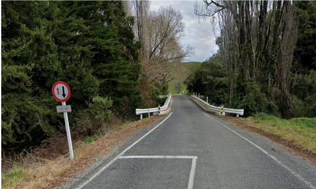
Figure No. 5.2 – Bridge 7: Te Anga Road (Source: Google Earth)
